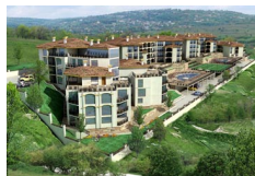
Kranevo Paradise Gardens 2, Kranevo
