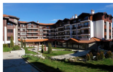
Mountain residence 7, Banskó
