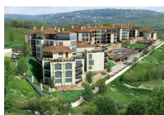
Kranevo Paradise Gardens 2, Kranevo
