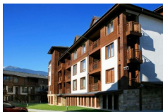
Adeona Residence, Bansko
