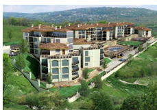
Kranevo Paradise Gardens 2, Kranevo
